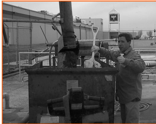
Tim Bowser works on converting hog-slaughter byproducts into a syngas which can be used to co-generate electricity and improve plant sanitation.
